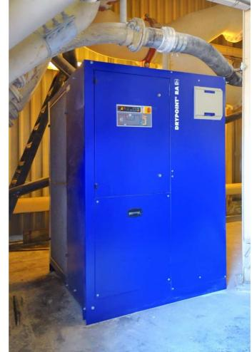
heat exchanger when entering the refrigeration dryer. Through this, the cooling performance of the refrigerant, which is required in the following air-refrigerant heat exchanger, is reduced and the system is particularly energy-efficient.
