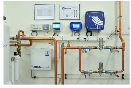
METPOINT MMA continuously records and monitors all of the decisive parameters in the central breathing air supply. The values that are recorded are the oxygen, carbon monoxide, carbon dioxide, sulphur dioxide, nitrogen oxide, and water vapour content.
