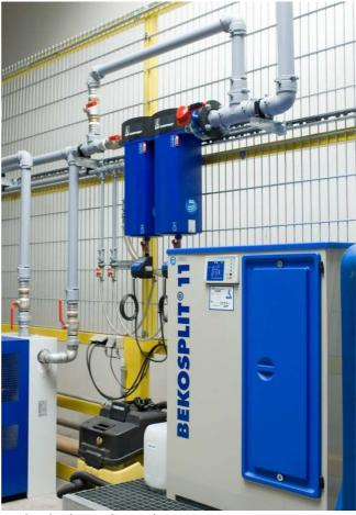
from impurities, the outflowing water can now be discharged into the wastewater system.
