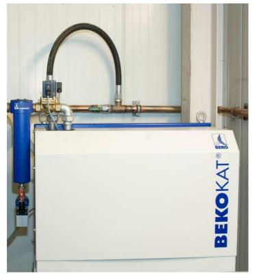
With the BEKOKAT method, it is for the first time possible to constantly achieve absolutely oil-free compressed air with a barely measurable maximum residual-oil content of 0.003 milligram per cubic meter of compressed air. This is the quality required in the most demanding fields of medicine, pharmaceutics, food processing and food packaging.
