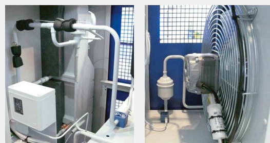
Internal view of a coated refrigeration dryer
